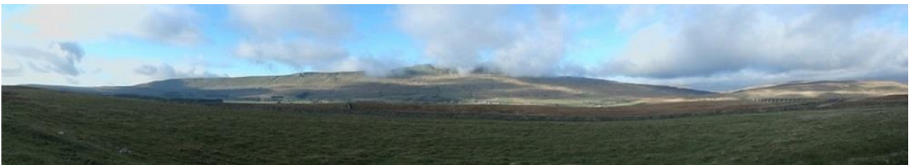
Whernside and Batty Moss viaduct – looking west and north from the cairn Photo: Yvonne Luke
