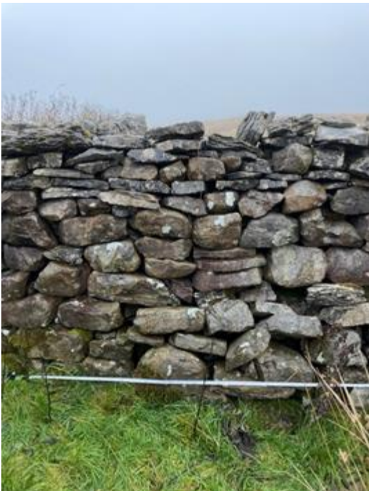
Photograph of a small section of the Sleights Pasture field wall boundary showing an intermixture of sandstone and limestone.
