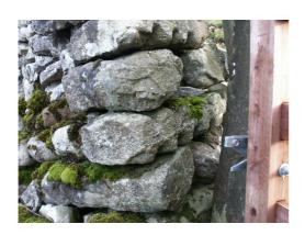
Fig. 13 Wallhead reusing corn drying joists
